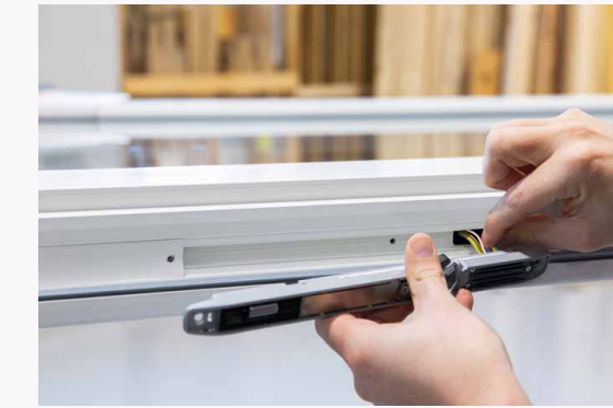
2: Attach the locking component and insert into the eurogroove
