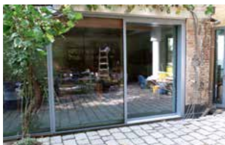
Assembly on the construction site
